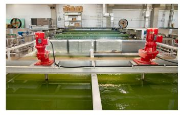
highly effective for cyanobacteria and algae related turbidity. Bubbles from the dissolution forces the organisms to the top of the water column, where they are skimmed off the top of the tanks. This projects benefits provide a sustainable solution to keep the public safe and to mitigate in-plant cyanobacteria challenges.
