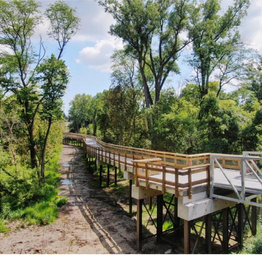
Metroparks Toledo selected DGL to design two access features that would allow visitors to the Swan Creek Preserve the ability to venture further into nature. The Connector Trail consists of a multi-use path, pedestrian bridge over Swan Creek, and an elevated concrete boardwalk through a mature tree canopy above the floodplain. Visitors can experience a unique perspective of the park, while not disturbing the wildlife below.
