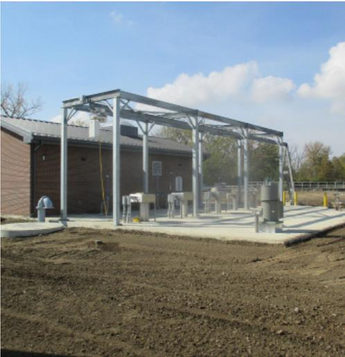
In Lebanon, Ohio, 80% of the city’s wastewater flow is received by the Glosser Road Pump Station and pumped five miles through a force main to the wastewater treatment plant. Due to the pumping distance, the 60-year-old pump station could not accommodate large wet weather events. After four overflows that discharged millions of gallons of sewage to a National Scenic River tributary within a two-year period, the Ohio EPA issued a Notice of Violation to eliminate future discharges.
