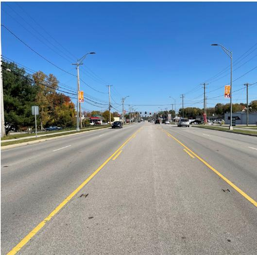
Engineering Associates completed the design of the LOR-20-22.13 - Center Ridge Road project which runs 2.3 miles through the core business corridor of North Ridgeville. The project widened the roadway from three lanes to five lanes and added sidewalks and a multi-use path to reduce accidents, relieve congestion, and improve pedestrian/bicycle safety.
